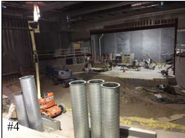
Photo #4 gives view of the auditorium when entering at street level on Highway 59. There is 10,000 square feet of new space which will seat 550.
