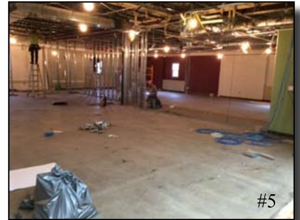
Photo #5 shows inside the science classroom demoed areas where asbestos abatement is completed and stud walls are going up.
